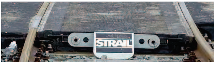
Figure 7 – veloStrail installation at a level crossing
