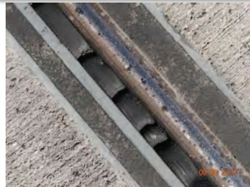
Zurich filler – breaking up
