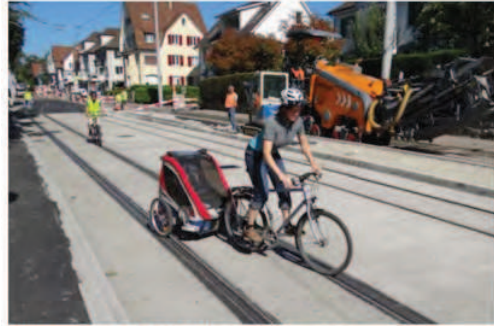
Test run on the cycle-friendly tram tracks
