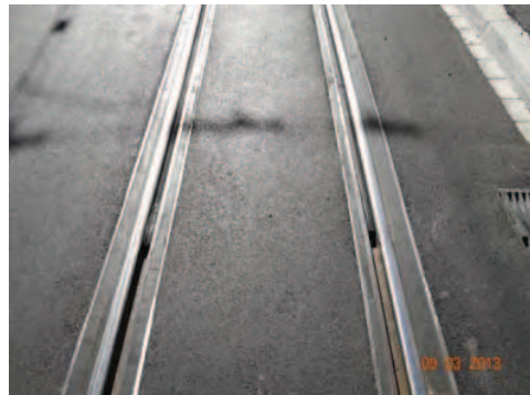
Zurich filler – stripping out
