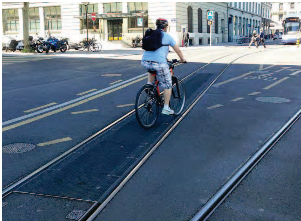
Figure 9 – short veloStrail insert section across a cycle lane - Geneva
