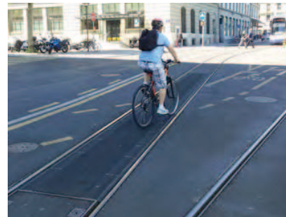
Short section of veloStrail – across a cycle lane - Geneva
